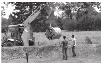
→ unloading: strap passed through the spindle
