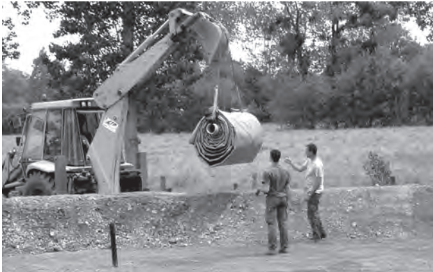
→ unloading: strap passed through the spindle
