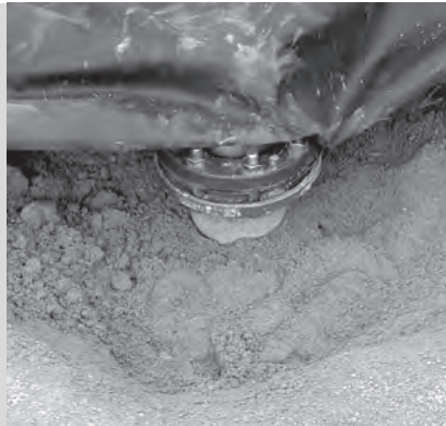
→ completed water-tight fitting
