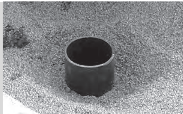
→ view of the pipe-work in place
